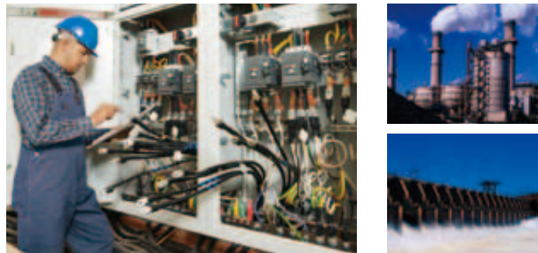
Supports high voltage systems around the world
